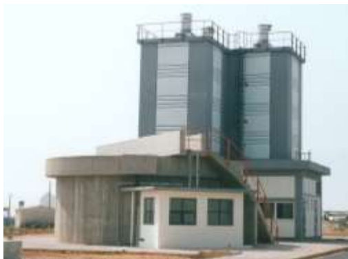
Water purification plant of Thessaloniki - Lime silo and Settlement tank
