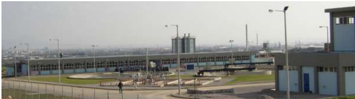
Water purification plant of Thessaloniki - Central unit of refinement
