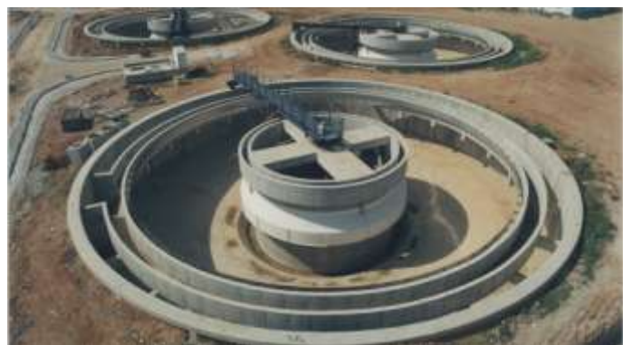
Water purification plant of Thessaloniki - Lime silo and Settlement tank
