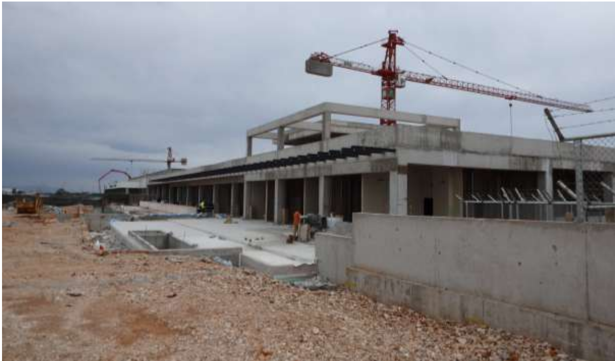
View of eastern extension of the main terminal during construction
