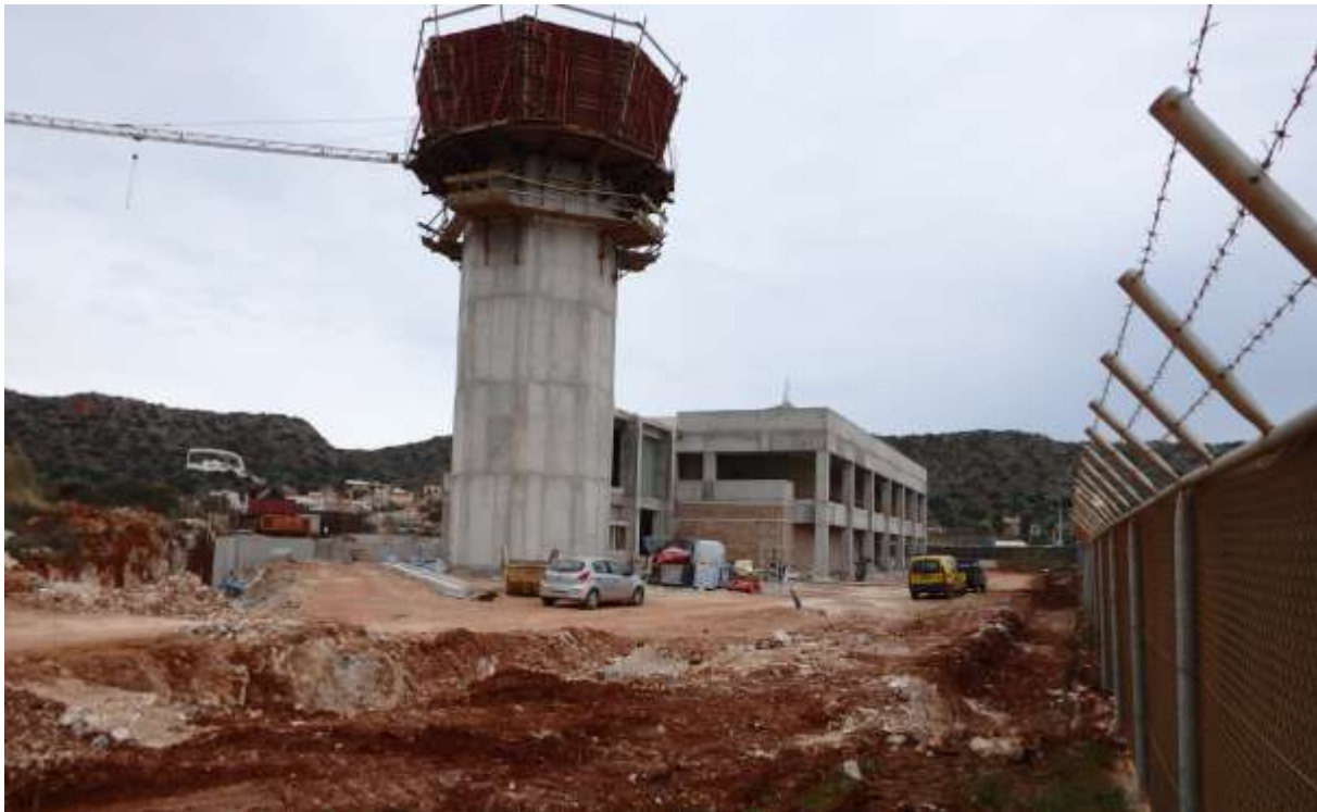
Control tower of Chania Airport during construction
