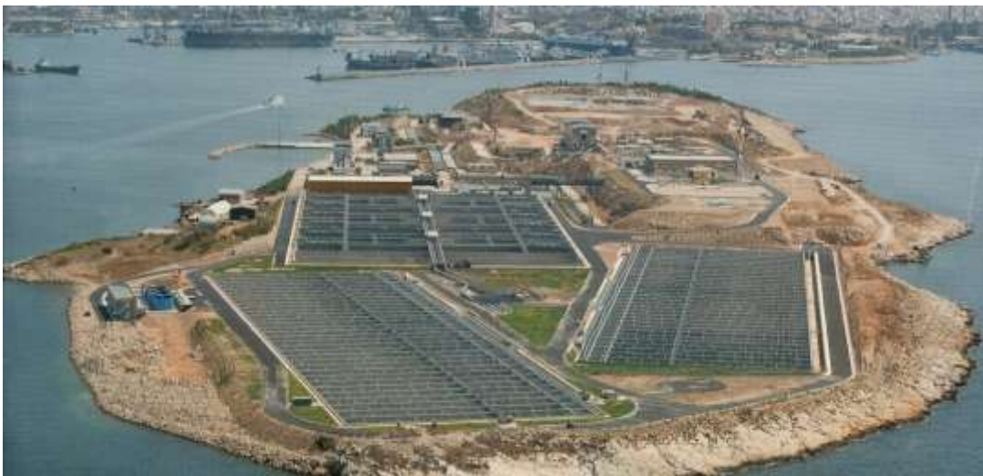
Overview of the wastewater treatment plant in Psyttaleia
