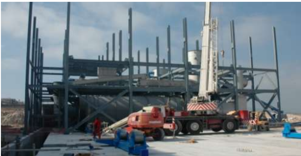
Sludge drying unit during construction
