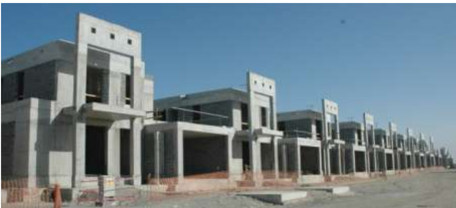
Villas under construction. Concrete works have been completed
