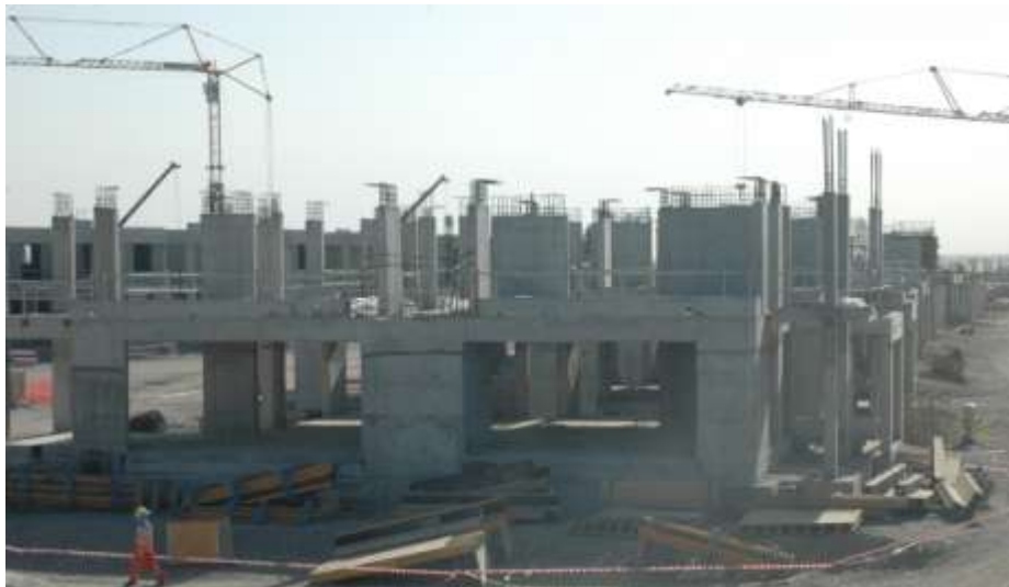
Apartment Buildings under construction
