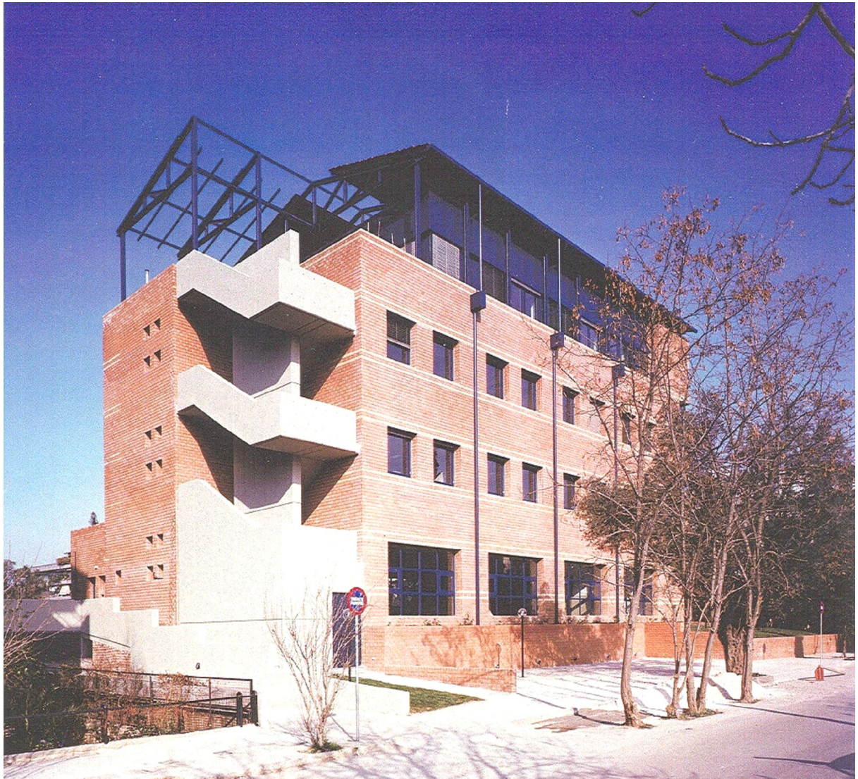
Office building of the Technical Company of Volos
