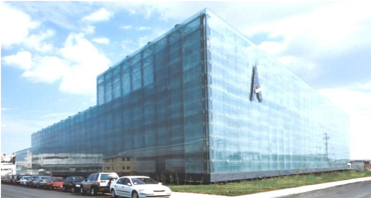
Office building complex of Alfa-Alfa Holdings: side facing Kifissos river
