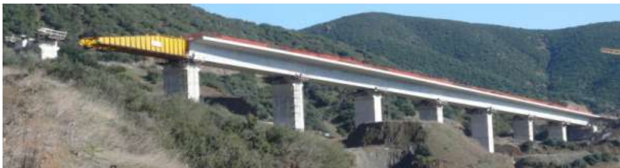
Bridges ΣΓ14 above and ΣΓ15 below, constructed with incremental launching
