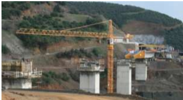
Bridge ΣΓ12, constructed with incremental launching. Top picture: the completed structure
