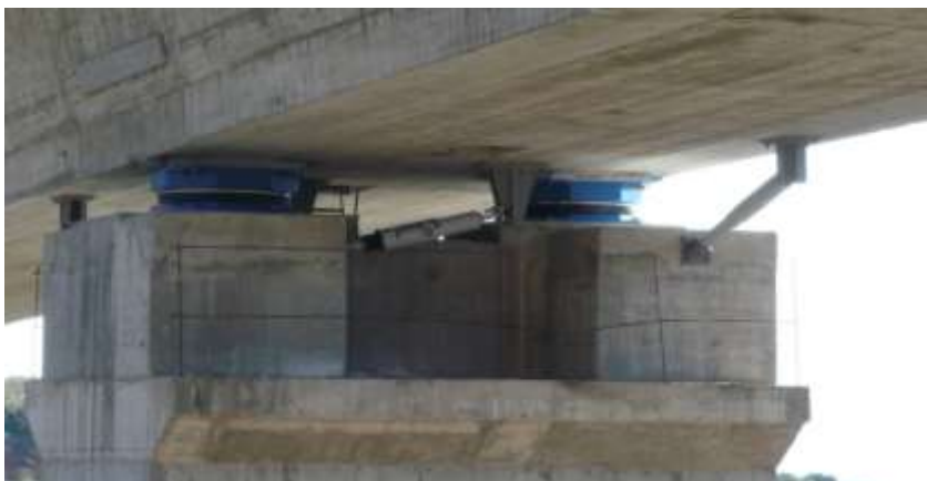
Detail of superstructure bearing on a pier depicting the seismic isolation devices
