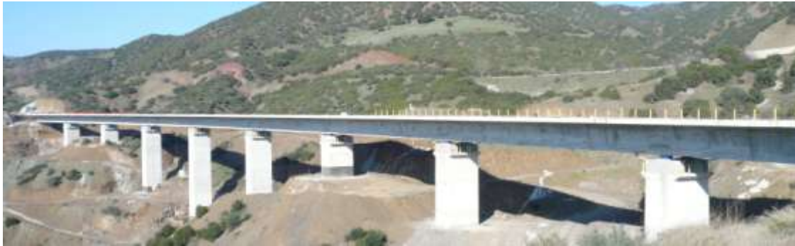
Bridges ΣΓ14 above and ΣΓ15 below, constructed with incremental launching
