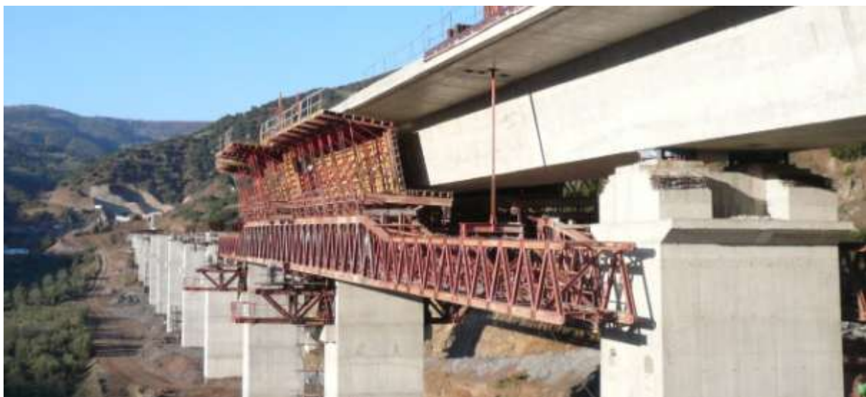
Bridge ΣΓ16, 660m long constructed with travelling formwork
