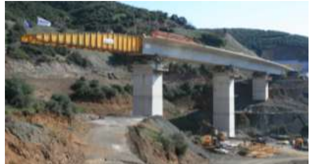
Bridge ΣΓ12, constructed with incremental launching. Top picture: the completed structure
