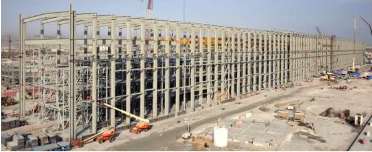
Exterior view of the ULD Building during steel erection phase
