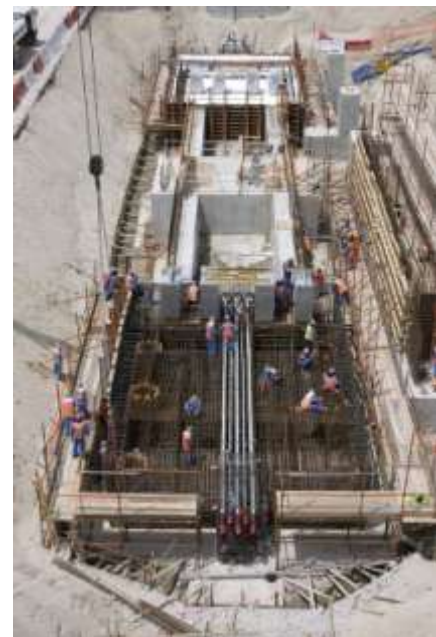
Front truss foundation with prestressing cables for the tie-beam
