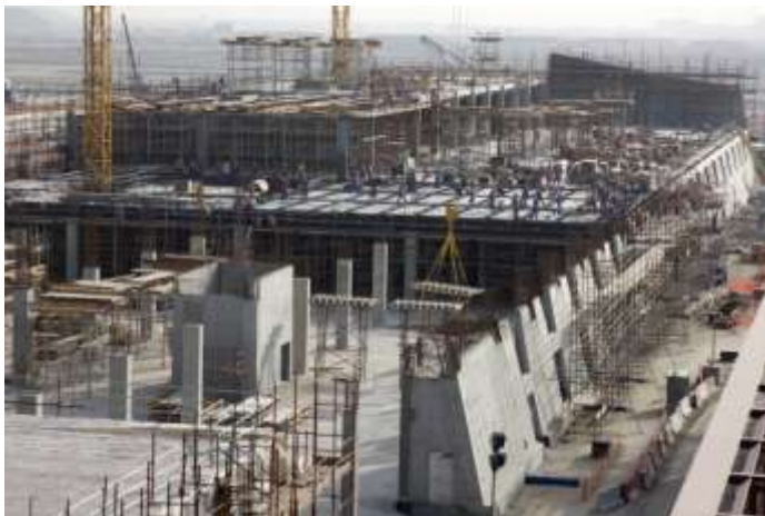
Construction of the Workshop Building
