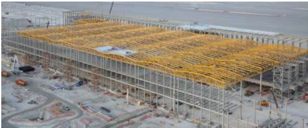
Exterior view of the Cargo Building during steel frame erection
