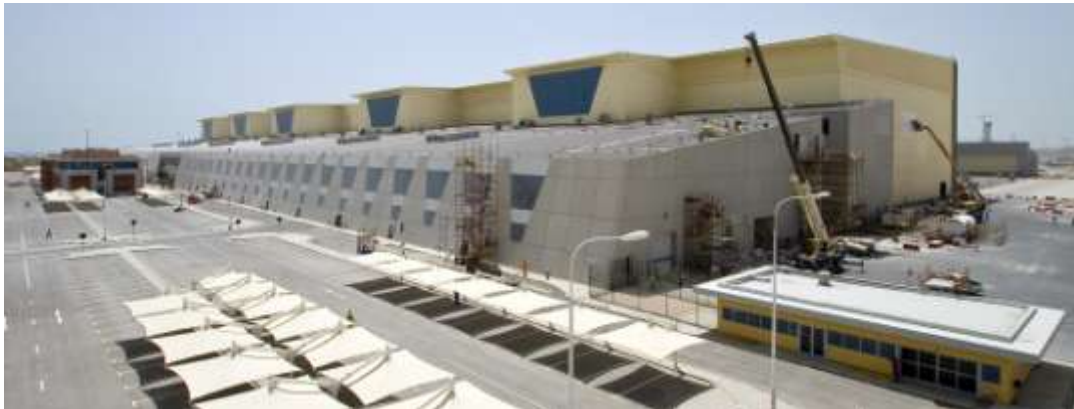
Front and rear view of the Aircraft Maintenance Hangar near completion
