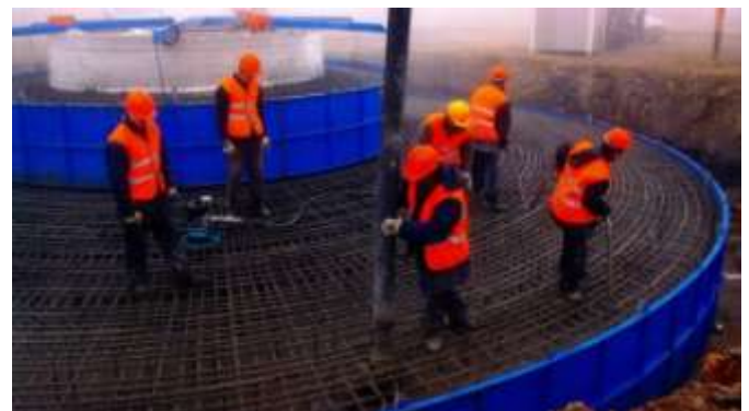
Construction of foundation for a 85m high Tower for ENERCON E70 wind Turbine
