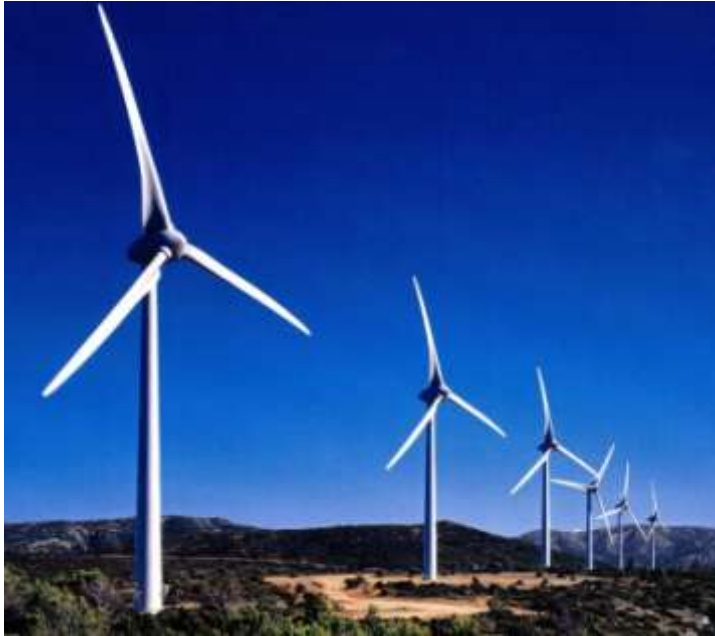
Wind park with ENERCON turbines
