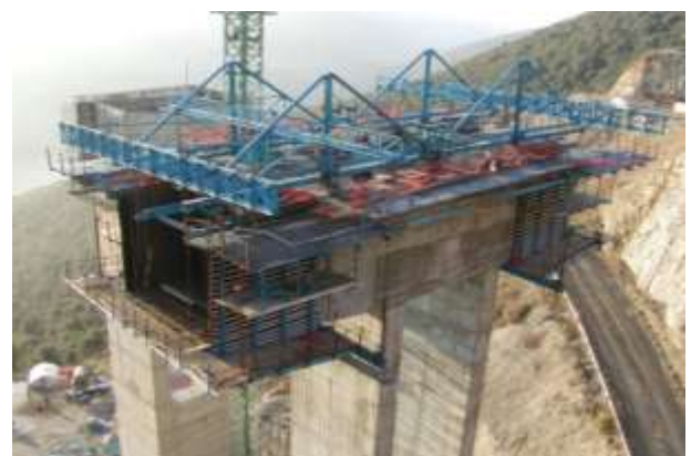
First construction phase of the deck segments
