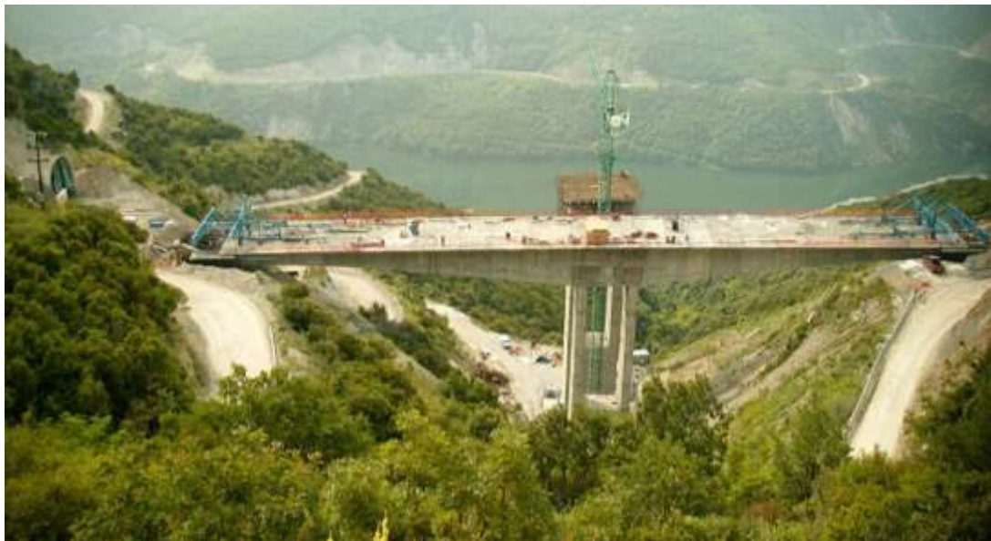
Construction of Bridge \Gamma 1 with the balanced cantilever method
