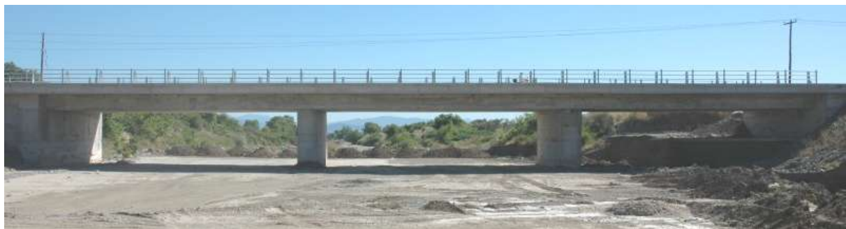
Bridge over Boagrio creek
