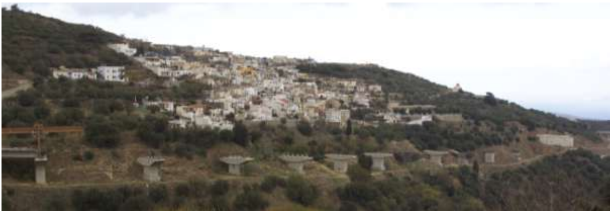
View of the previously constructed piers (part between M10 and M20)
