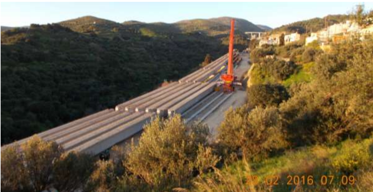
View of the precast beams
